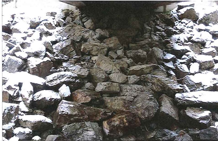
CK2278 Right Abutment
