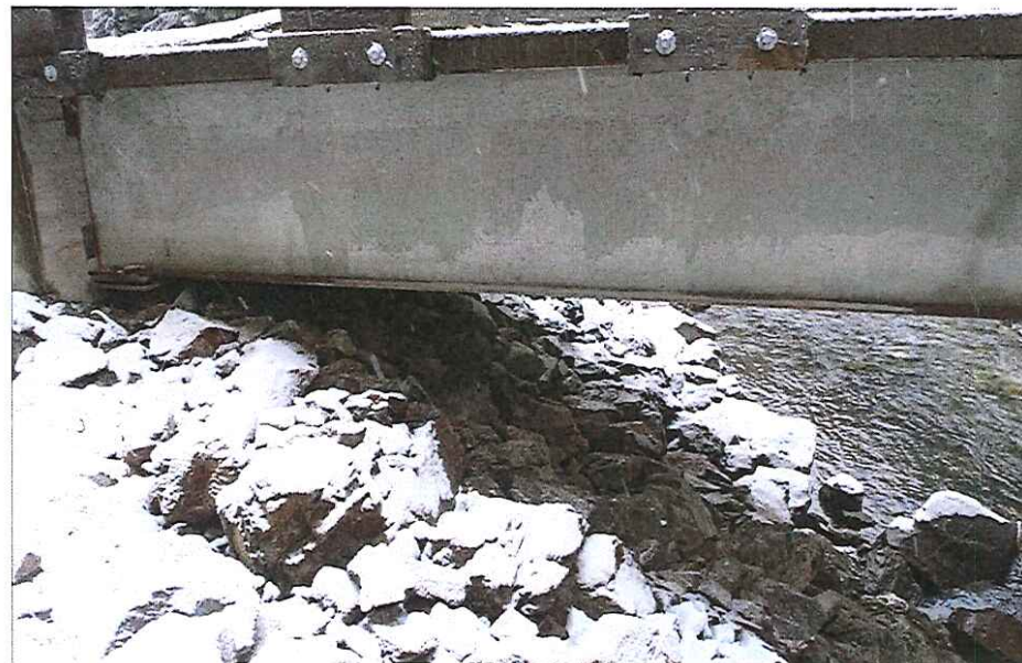
CK2278 Left Abutment Rip Rap
