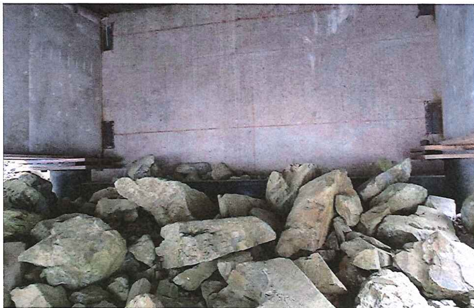
CK2278 Left Abutment
