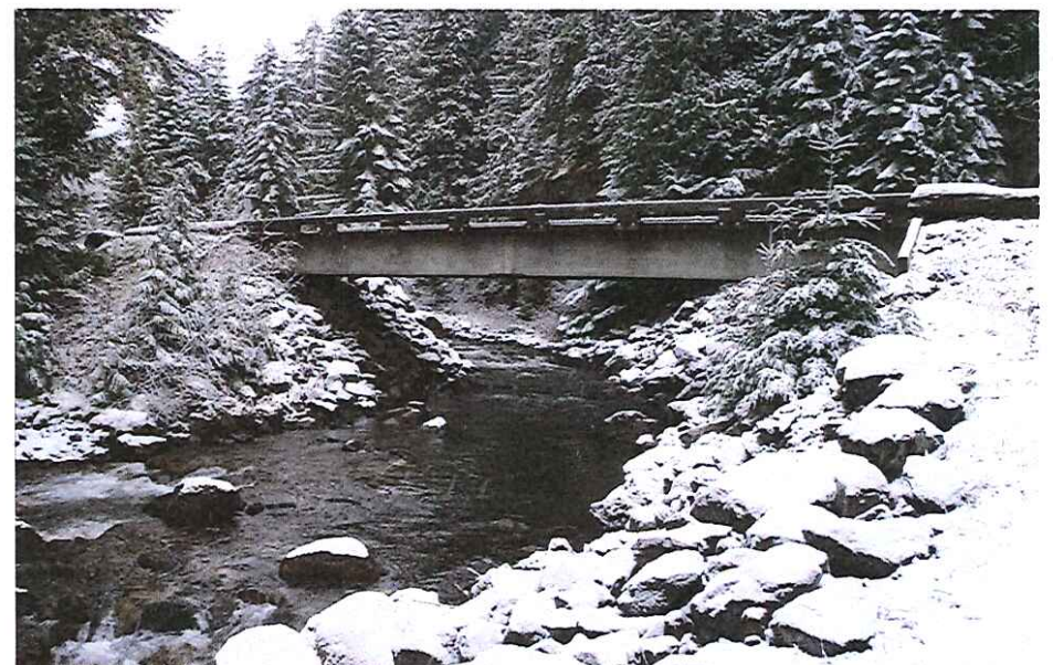
CK2278 From Downstream
